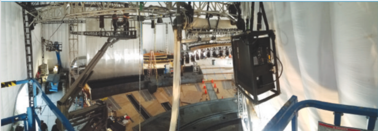
The installation in progress.
